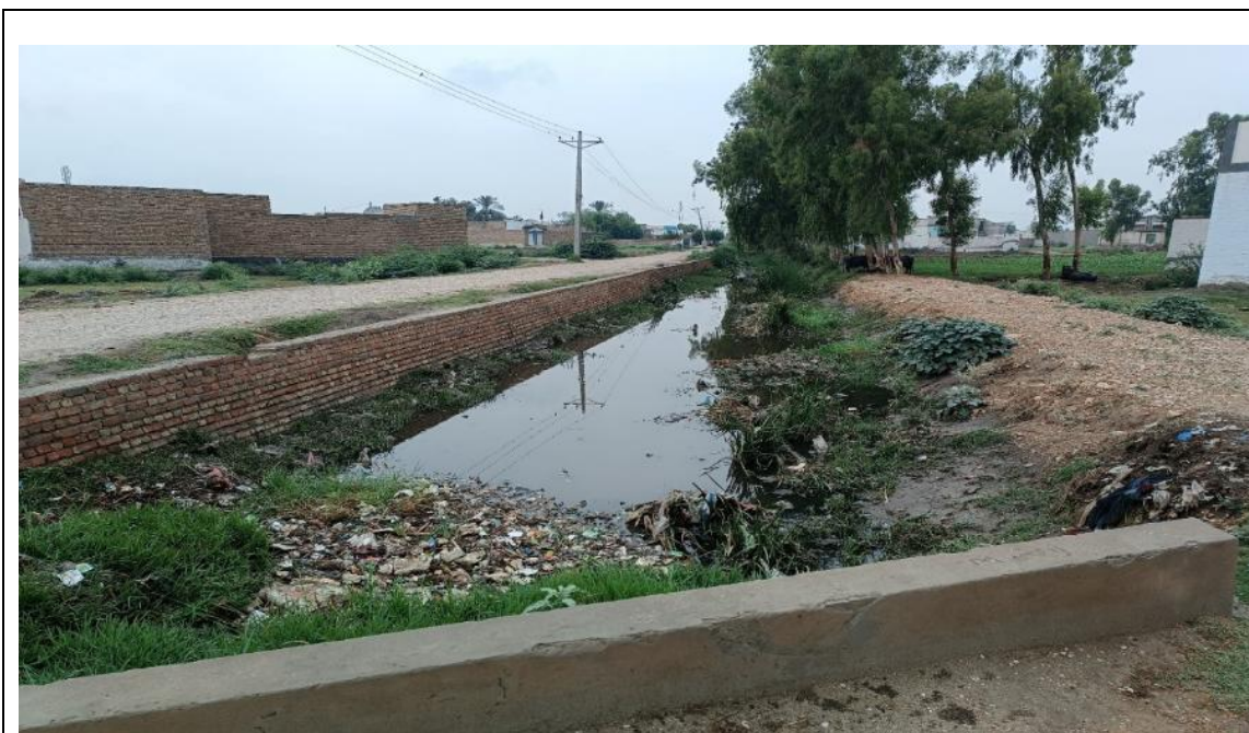
Figure 2.3: Brick Retaining Wall Side Protection
